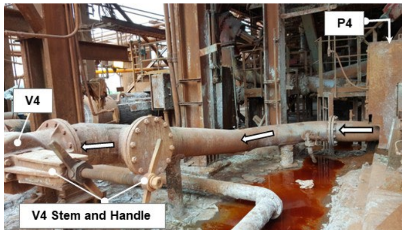
Figure 8. Undamaged #4 DBO Pump discharge piping and #4 Valve with flow direction arrows (for reference)
